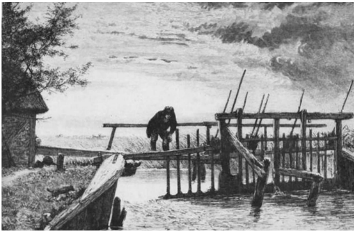
Fig. 10. Engraving of an upper Thames weir and flashlock.
