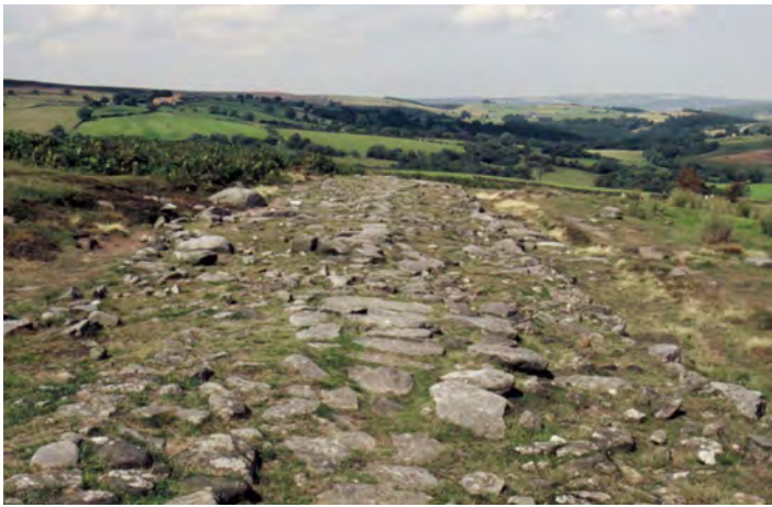
Fig. 6. A mile-long stretch of a probable Roman road crosses isolated moorland at Wheeldale, North Yorkshire. Its hardcore and drainage ditches can be seen.
