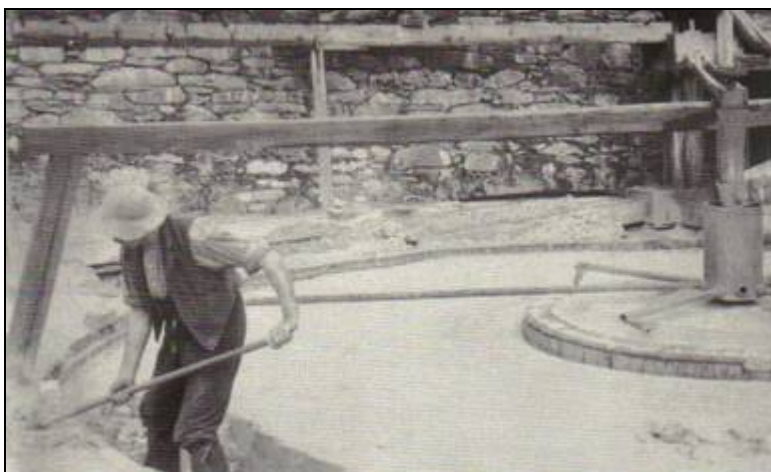
Illus. 11: Digging out the waste component of the buddling process from the outer part of the buddle pit.
