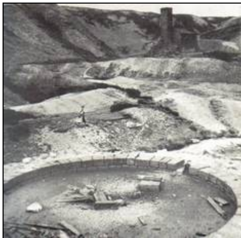
Illus. 13: An abandoned buddle with apparent traces of removed machinery and signs of a possible central hub support.
