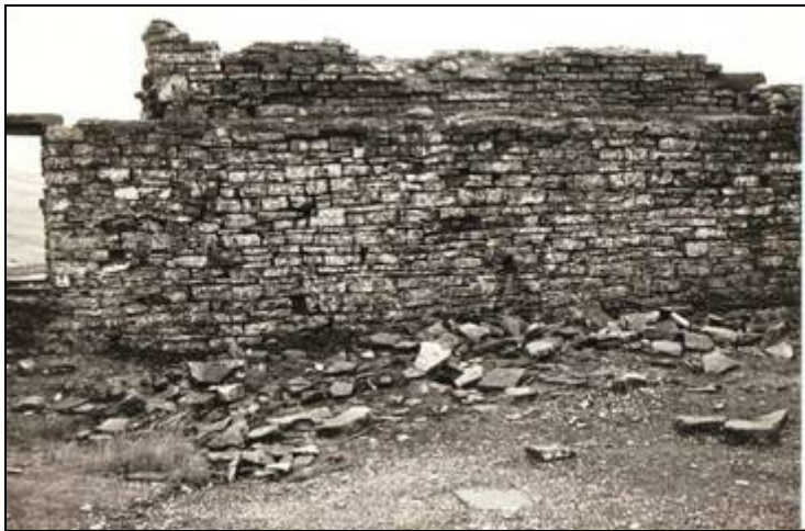
Illus. 14: Interior view of the north wall of the Buddle House prior to repair and reconstruction in the 1980s.
